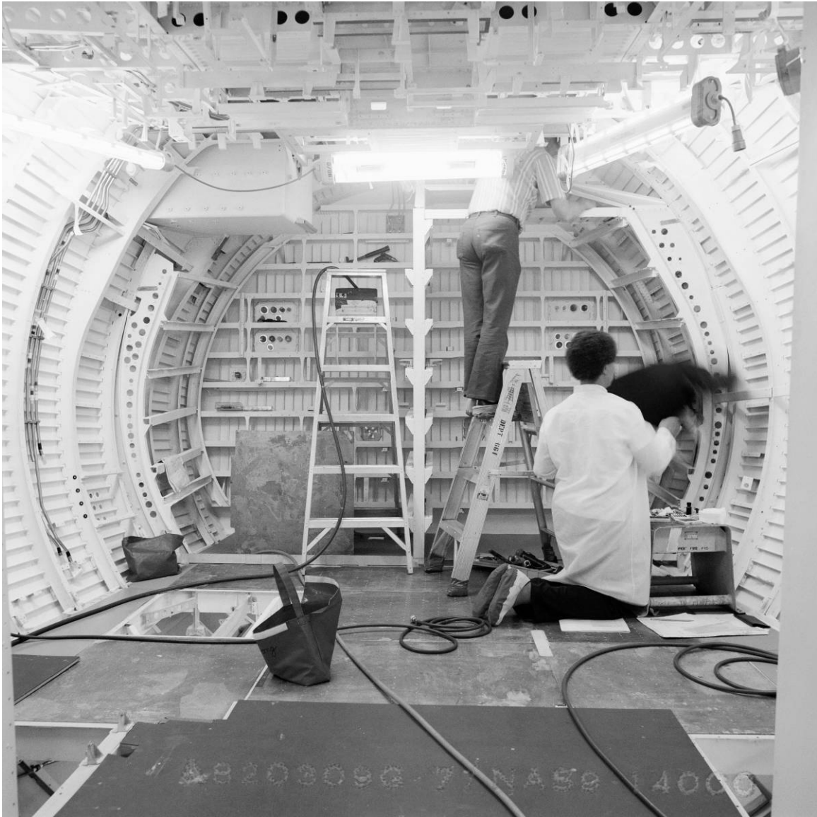
Figure B-11. Manufacturing operations on Discovery's middeck, NAR Building 290, Downey, California, March 9, 1982. Source: NASA, Johnson Space Center Image Repository, JSC2010-03244.
